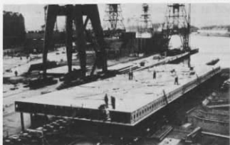
Commencement of building. First pre-fabrication laid at yard (Fairfield-Govan).
