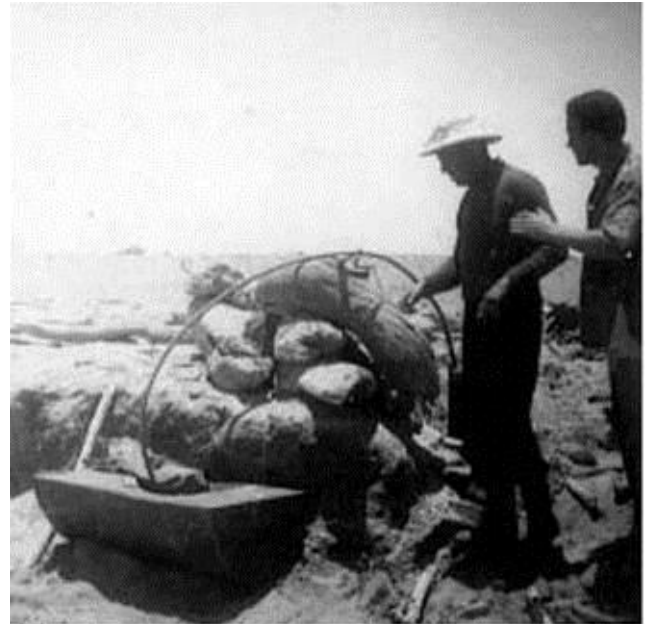
MR. LOUTITT, MATE & 2ND ENGR. J. NASH WITH WATER CONDENSOR. FUEL WAS DRIED UP TREES & DRIFTWOOD.
