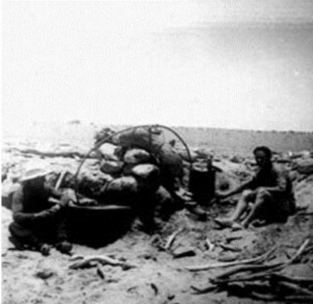
WATER CONDENSOR : SALT WATER IN TIN WITH FIRE UNDERNEATH, PIPE HAS HOLLOW DODGER STANCHION, BUCKET TO RECEIVE FRESH WATER STANDING IN A BUOYANCY TANK FULL OF WATER. ONE BUCKET OF WATER, SLIGHTLY BRACKISH, WAS OBTAINED ON FIRST DAY. 2ND. ENGR. IS TENDING FIRE & THE MATE IS BY THE TANK.
